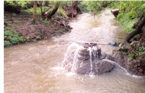
Sanitary Sewer Overflow - SSO
