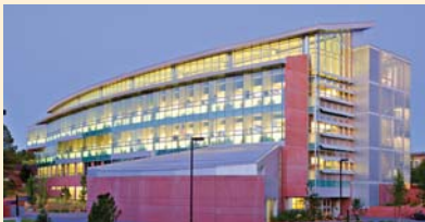
Project: Northern Arizona University College of Business Administration Client: Northern Arizona University Location: Flagstaff, Arizona
