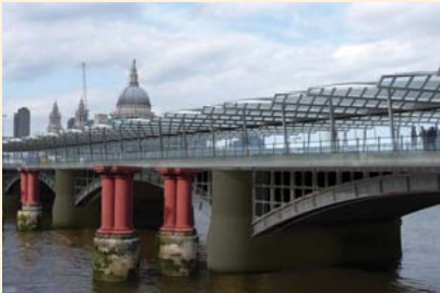
Project: Blackfriars Station and Bridge 410 Roof Client: Network Rail Location: London, England
